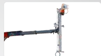
Spray painting operation
